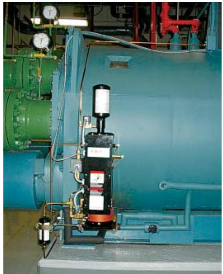
Debra-Kuempel (Cincinnati, OH) installed 3 OAM-Purgers on 3 high pressure refrigerant (R-12) centrifugal chillers located at Harbor Group Management Company's PNC Center in order to regain system capacity that was lost to oil entrained in the chillers refrigerant charge (these OAM-Purgers removed 9.5 gallons of excess oil in Chiller 1, 6 gallons of excess oil in Chiller 2, and 22 gallons of excess oil in Chiller 3).
