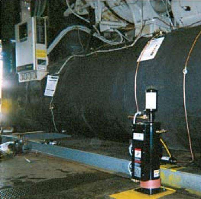
Joseph Davis Mechanical recognized oil entrained in a chiller's refrigerant charge at the 3M facility in Buffalo, NY. The OAM-Purger was recommended as a possible solution. The OAM-Purger regained system capacity and decreased energy usage.
