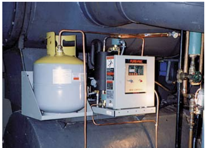
High-efficiency purge unit with optional carbon collection canister installed on an R-11 chiller in a hospital.
