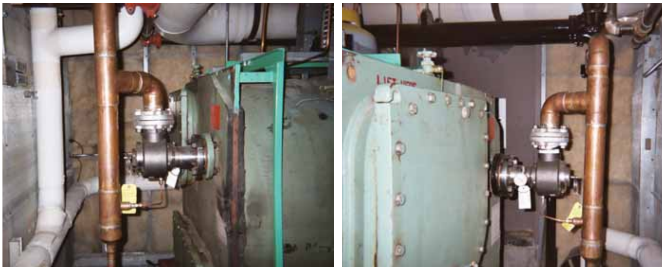
Photos are of the RuptureSeal Model NRS-2 backup safety relief valves for low pressure centrifugal chillers installed by Johnson Controls Alaska at the BP and Frontier Group facilities.
